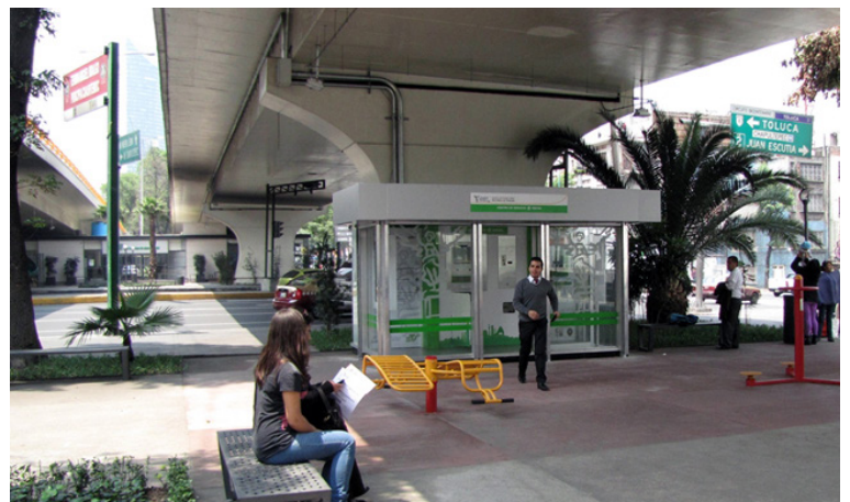
Bajos Puentes Underpass Program (2013), Mexico City MX
